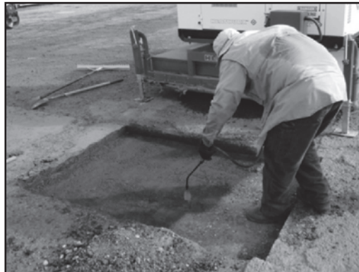
Figure A12. Rejuvenator applied to repair void.
