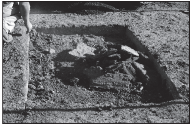
Figure 41. Squared edges and large chunks from saw cutting.
