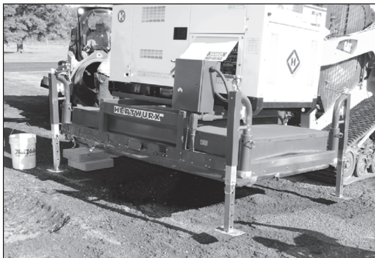
Figure A9. Heater placed over the rejuvenated stockpile.
