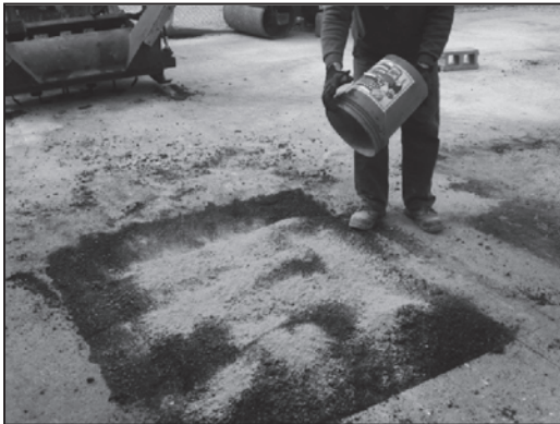
Figure 61. Cement addition to PHP-4.
