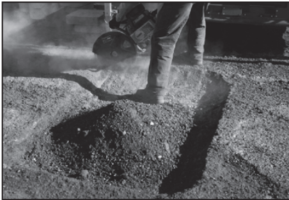
Figure 40. Squaring repair edge with saw.
