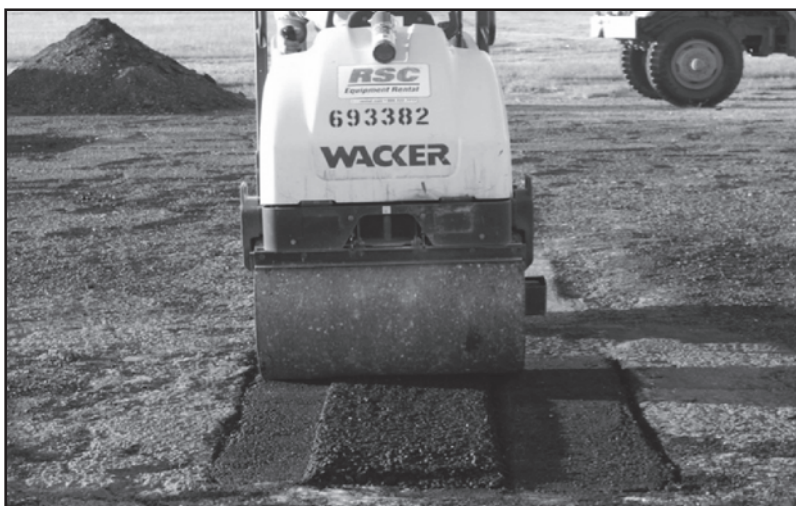
Figure A15. Compaction of final lift.
