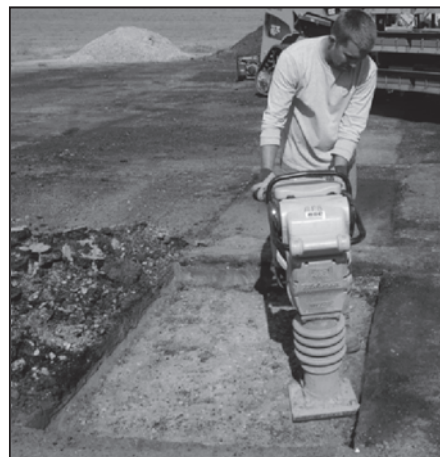
Figure 43. Base compaction (full-depth).
