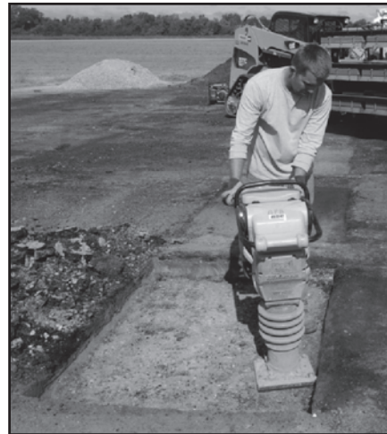
Figure A11. Base compaction for full-depth repair.
