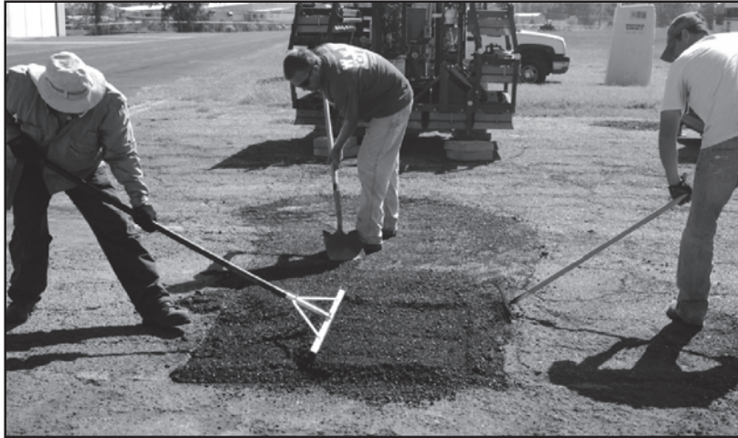
Figure A14. Preparing final lift for compaction.
