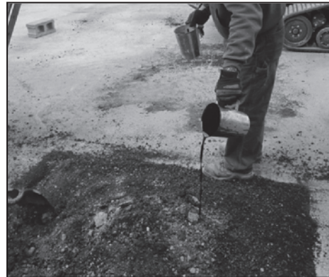
Figure 62. Rejuvenator addition to PHP-4.
