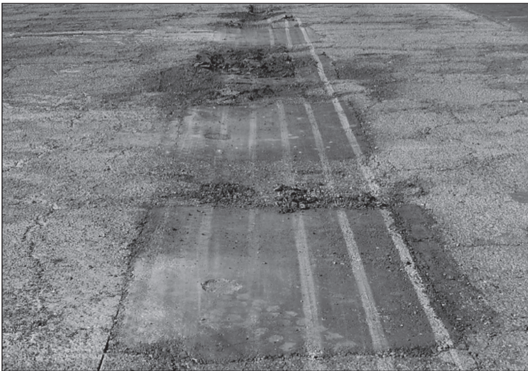
Figure 67. Partial-depth repairs lane after traffic (front to back: PD-4, PD-3, PD-2 and FD-1a).
