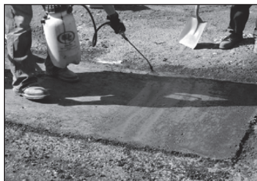
Figure 56. Typical rejuvenator application to mitigate surface cracking.
