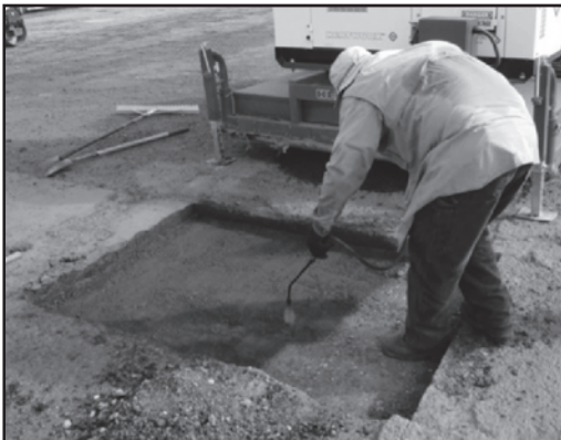
Figure 44. Rejuvenator applied to repair void.
