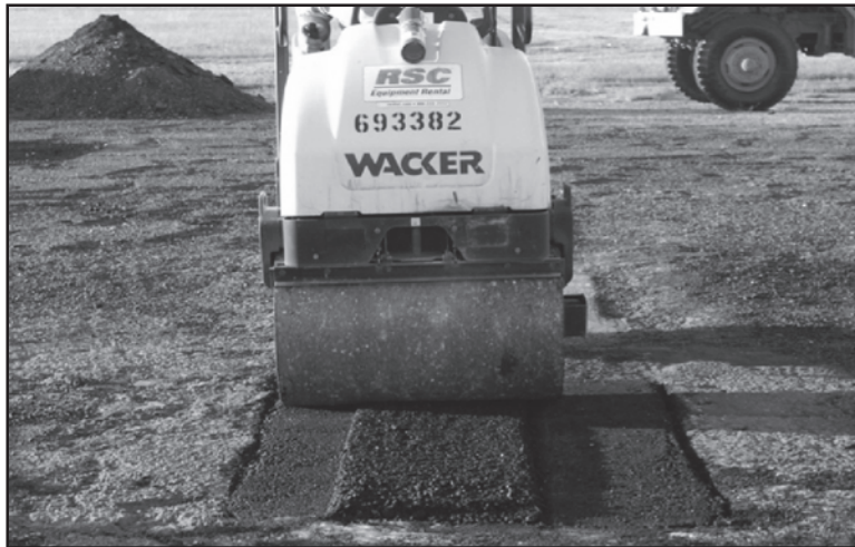
Figure 51. Dual-drum compactor pinching edges of repair.
