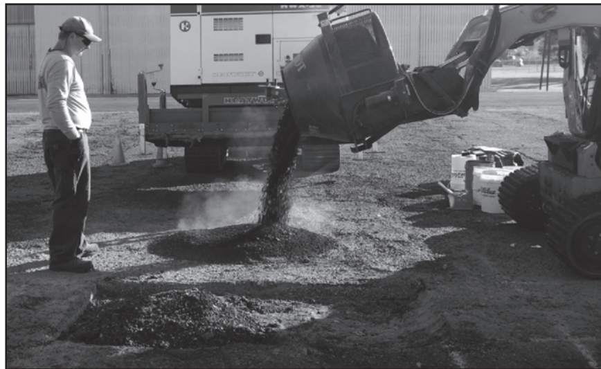
Figure 48. Rejuvenated asphalt being stockpiled near repair.
