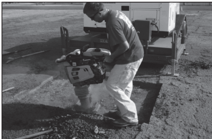
Figure 30. Base material being compacted.
