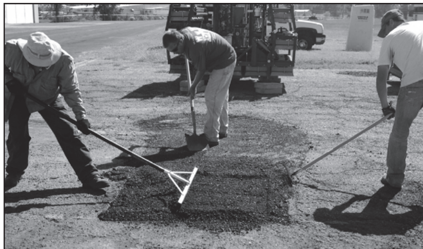
Figure 50. Rejuvenated material being prepared for compaction.
