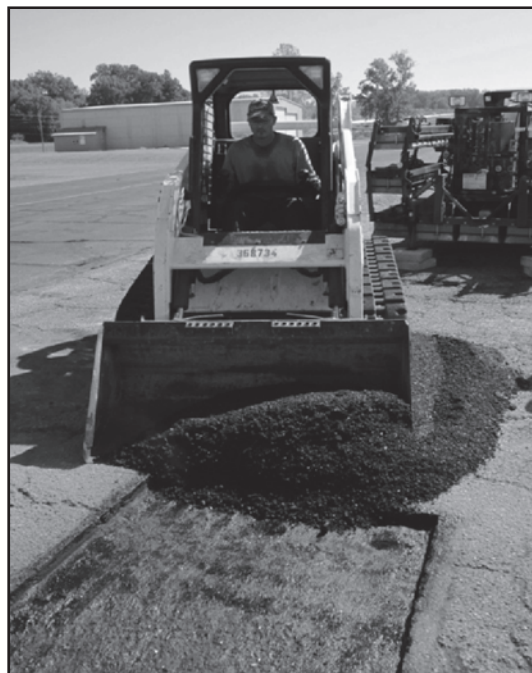
Figure 49. Rejuvenated stockpile being placed into repair void.
