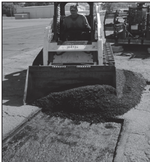
Figure A13. CTL placing rejuvenated material into repair void.
