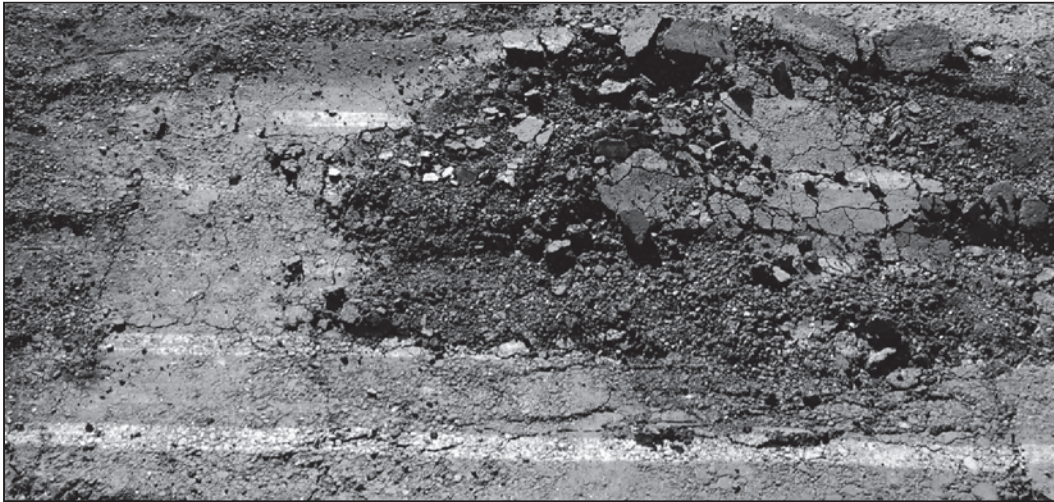
Figure 70. Repair PD-2 after traffic.
