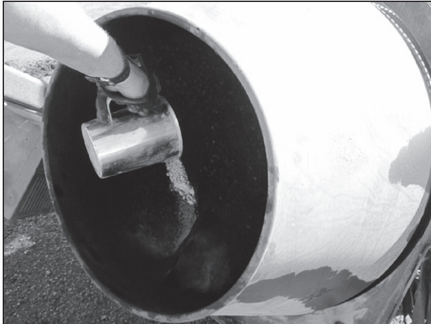
Figure 46. Cement being added to rejuvenated batch mixture.
