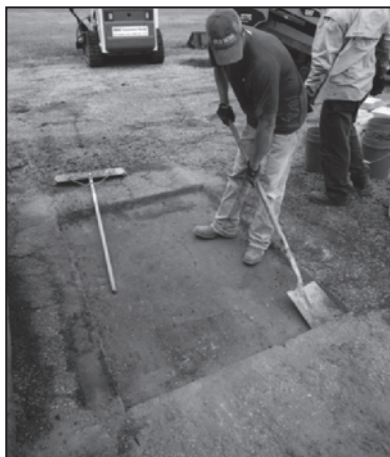
Figure 42. Final repair void preparation (partial-depth).
