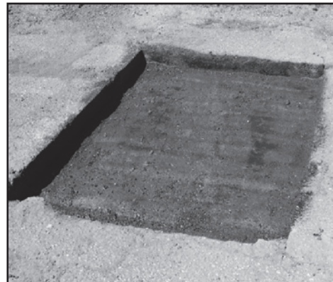
Figure 45. Repair prior to asphalt placement
