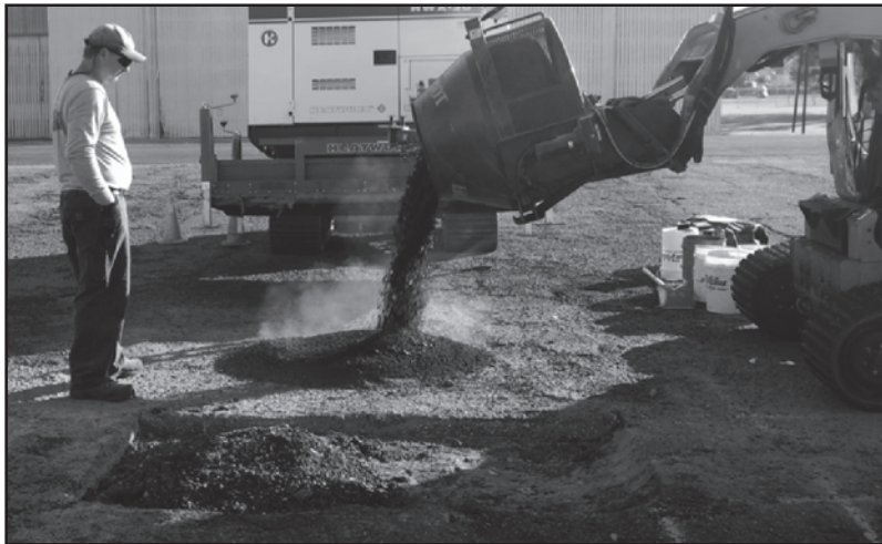
Figure A8. Rejuvenated asphalt being stockpiled near repair.
