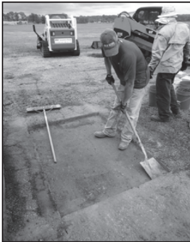
Figure A10. Final repair void preparation for partial-depth repair.
